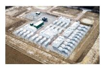
This project is designed to absorb or output up to 132 megawatts of electricity and will consist of several battery storage containers with associated on-site additional support facilities consisting of a project collector substation, inverters, collector lines, fencing, access roads, operations and maintenance building, supervisory control, a SCADA system and other ancillary facilities or equipment. The project also includes a 115-kV overhead gen-tie line, which would extend to the
